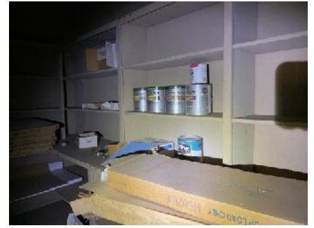
Example of stored materials including paints and cleaning products
