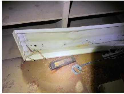
Example of standard fluorescent light fixture including 2 bulbs and one possible PCB containing ballast
