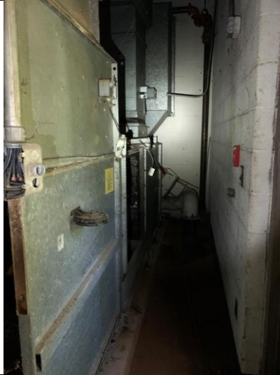
Air handler at back of boiler room, no suspect materials present
