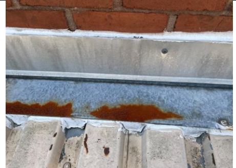
Roofing caulk tested negative for asbestos at metal awning
